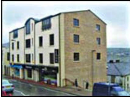
Fountain House is geothermally heated and cooled. Photo courtesy of www.news.bbc.co.uk
